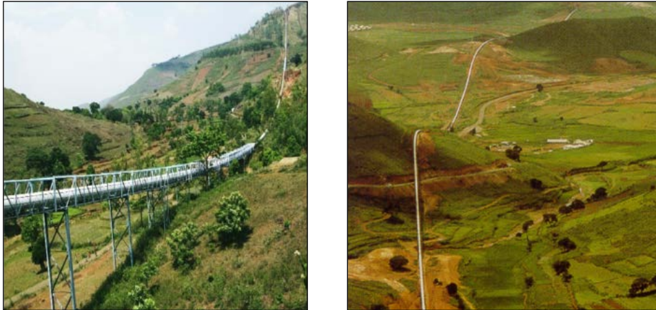
Fig. 4.9: Cable belt conveyor; Asia's longest (14.6 km) single flight multi-curve cable belt conveyor Courtesy: Panchpatmali (C&N Block) Bauxite Mine of M/s NALCO
