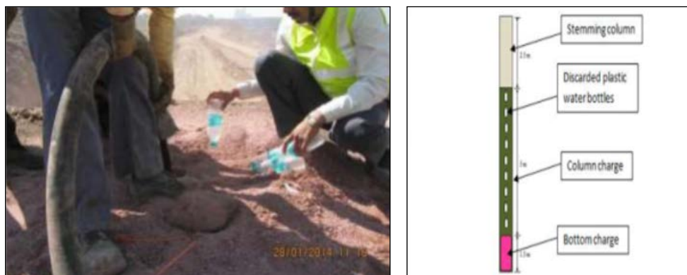
Fig. 2.16: Spacer for blast hole and blast hole cross section
